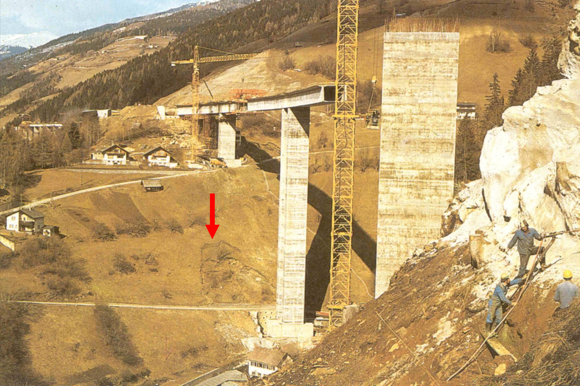
Sliding mass creeps aside the protective shell
