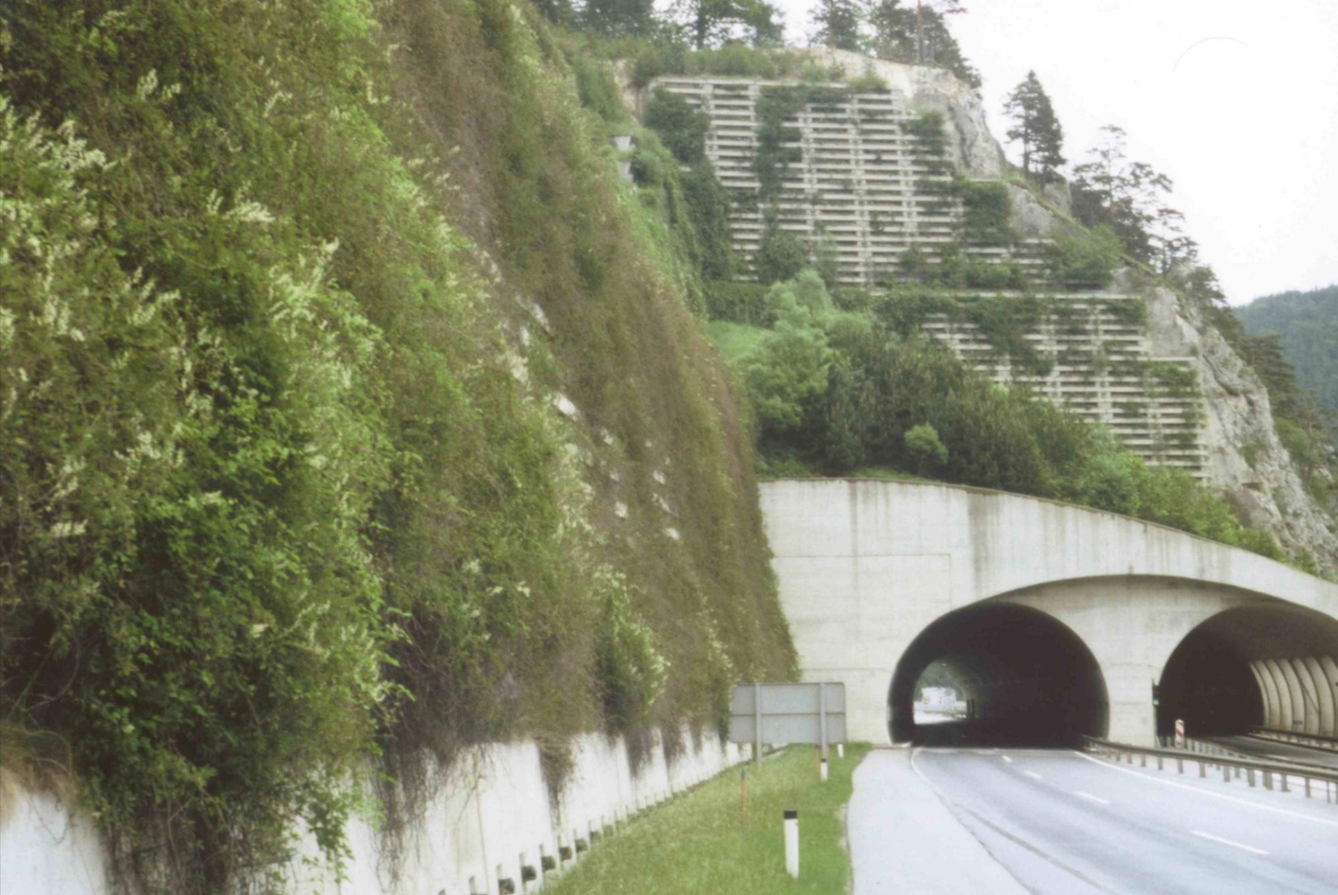
Crib walls of max. 43m height (locally tied back)
