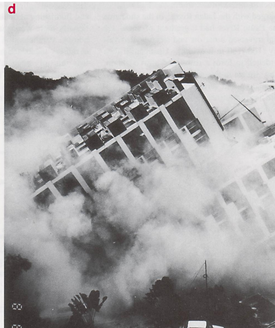
HIGHLAND TOWER (Kuala Lumpur) Collapse due to sliding slope
