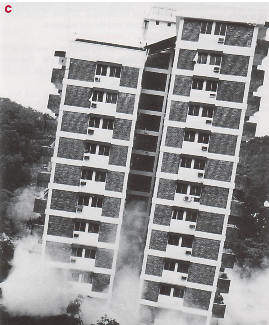
HIGHLAND TOWER (Kuala Lumpur) Collapse due to sliding slope
